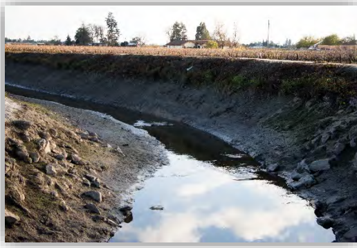
Figure 1 - Channels, streams, and drainage ways are over taxed by increases in runoff caused by increased development and impervious surfaces.
