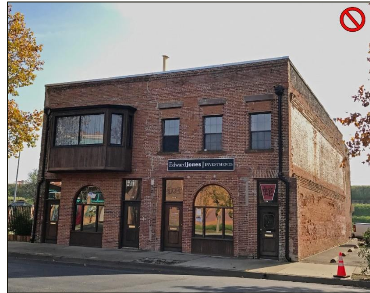
Figure 8. The second-story wood-sheathed bay window negatively impacts the historic character of the building and smaller than the original replacement windows installed in the upper story, non-historic reflective coatings on windows applied (not permitted)
