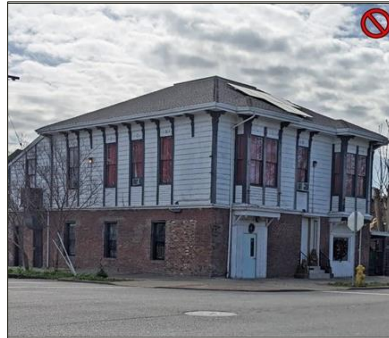
Figure 11. Solar panels mounted on the primary elevation of a historic building (not permitted)
