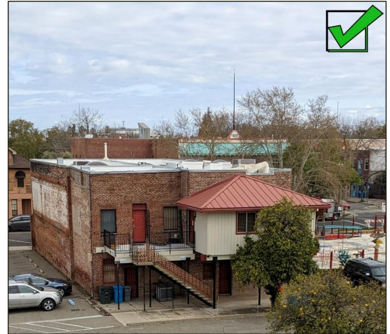
Figure 1413. The addition to 310 1st Street was constructed on a secondary (rear) elevation and smaller in size and scale to the historic building and not visible from the public right-of-way
