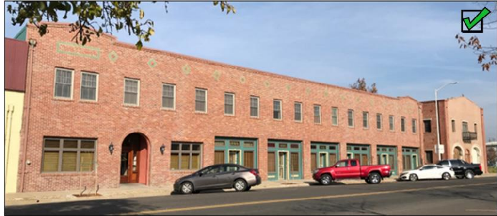
Figure 6. Historic masonry is retained on Third Street
