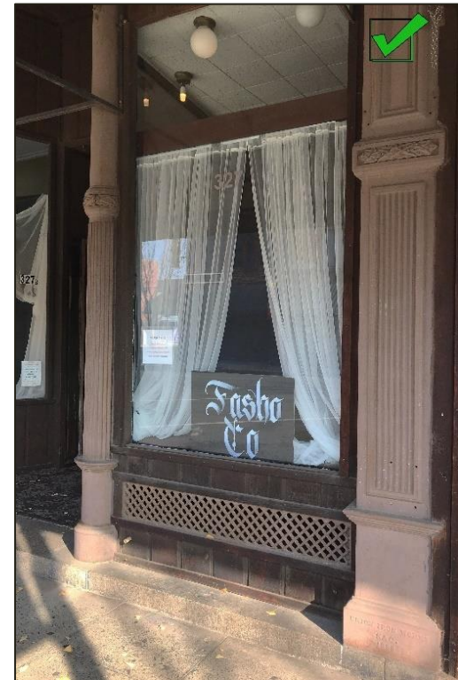
Figure 4. Character-defining original cast iron storefront has been retained
