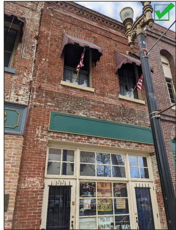
Figure 10. Awnings are placed over upper-story windows and are made from materials and designs that match those used historically
