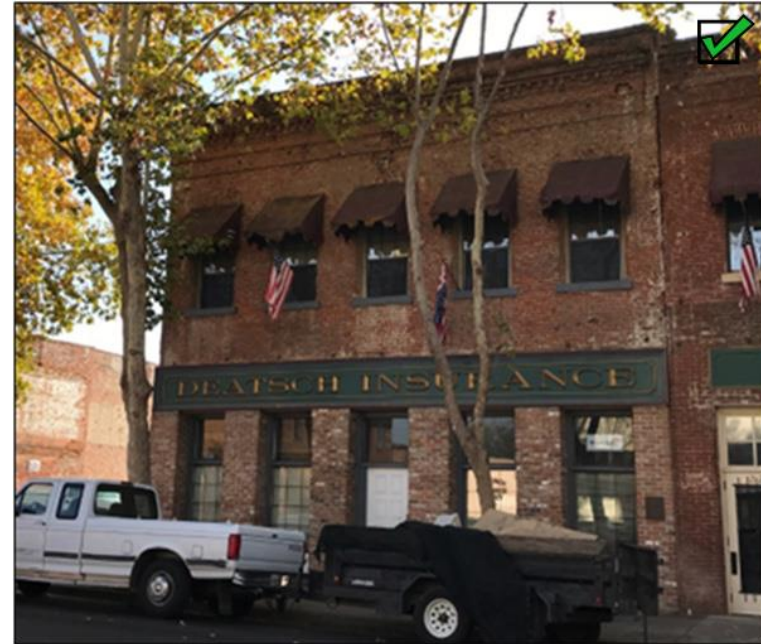
Figure 9. Retained historic commercial storefront on First Street
