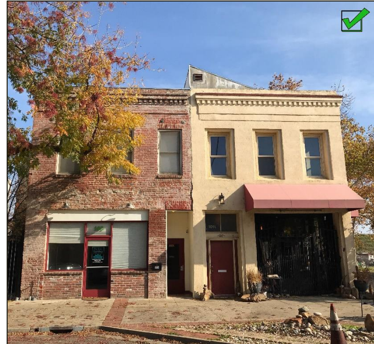
Figure 1312. 101 and 103 C Street retaining the historic zero-foot setback from the sidewalk
